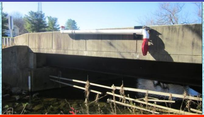
This dry hydrant installation is mounted to a jersey wall-type bridge wall over a local creek. The installation uses a saddle-mount design that "slips" over the concrete wall and is held in place by friction and tension bolts without drilling any holes into the bridge. The design minimizes exposure to snow plows and vandalism.
