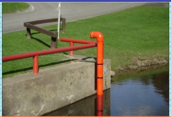
This wall mount installation used a GBW saddle mount bracket on the concrete wall to hold the standpipe in a "fixed" location. No holes were drilled in the wall, which also allows for repositioning the standpipe if needed over time due to changes in the lake bed.
