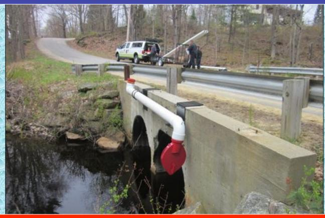
This bridge-mount was installed on a Town-owned bridge and used the GBW saddle mount system of attachment. No holes were drilled into the concrete bridge structure.
