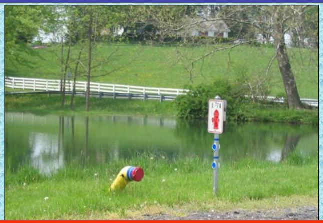
This 6-inch dry hydrant had developed an air leak and was repaired by GBW Associates, LLC by replacing the 45-degree elbow and installing a new 6-inch NST male suction head.
