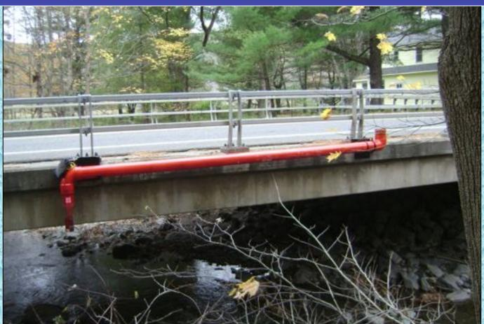
This standpipe was installed on a State-owned bridge and was the first GBW installation where the brackets were bolted to the bridge.
