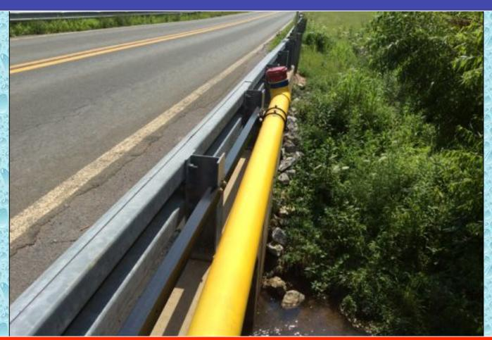
The system attaches directly to the guard rail posts and the brackets are adjustable to allow for stream flow changes over time.
