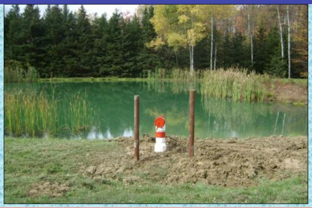
This traditional installation used 20-feet of 8-inch PVC pipe outfitted with a barrel strainer. The pipe was then reduced to 6 inches at the full-time swivel and then trimmed out with a 6-inch NST male suction head.
