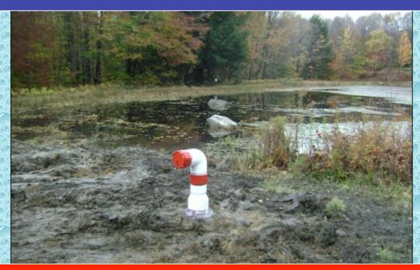
This traditional dry hydrant was installed in a pond in the Alleghany National Forest. Forty-feet of 8" PVC pipe was used to get the 8" barrel strainer far enough out into the pond to be away from aquatic growth. The 8" pipe was reduced to 6-inch pipe at grade level and then trimmed out with a 6-inch NST male suction head connected to a full-time swivel.
