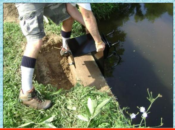
Saddle mount brackets were used for this installation. No holes were drilled into the concrete bridge abutment.
