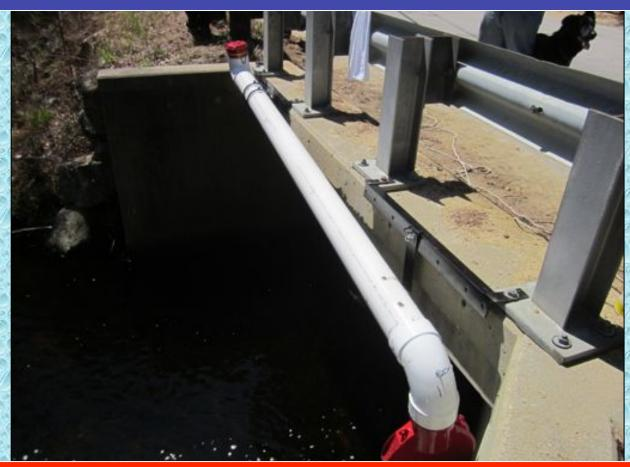
The installation used the angle mount brackets that were bolted to the bases of the guardrail posts using the existing bolts.
