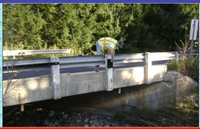
The bridge had wooden guardrail posts. The DFH mounting system used the existing bolt holes in the posts; however, each bolt was replaced with a new, galvanized bolt.
