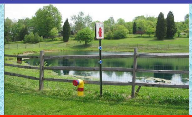
This traditional dry hydrant was installed by GBW Associates, LLC in a pond at a local nursing home. The 6-inch PVC pipe was outfitted with a tear drop style suction strainer and the 6-inch NST male suction head was connected to a full-time swivel.
