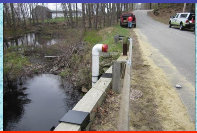
Once deployed, the suction head is in position for access by the FD pumper.
