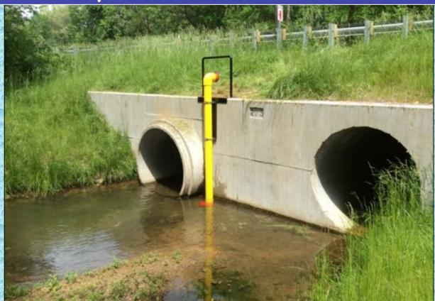
This installation used a modified, saddle mount bracket to secure the standpipe. No holes were drilled into the concrete wall.
