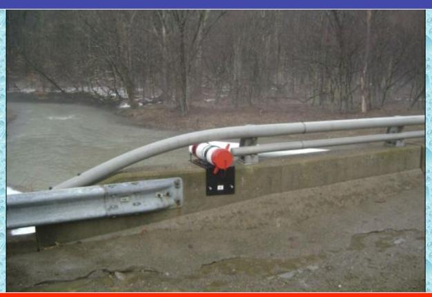
This bridge-mounted installation used a 20-ft articulating arm outfitted with a teardrop strainer to reach the water below. The articulating arm was used because of the limitations created by the guardrail.
