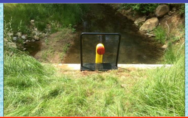
A 2" steel pipe safety railing was added due to the location of the suction head and lack of bridge railing or guardrail.
