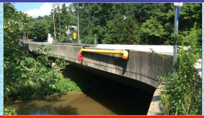
This dry hydrant installation is mounted to a "jersey" wall type of bridge over a local river. The installation uses a saddle-mount design that "slips" over the concrete wall and is held in place by friction and tension bolts. No holes are drilled into the bridge. The design minimizes exposure to snow plows and vandalism.
