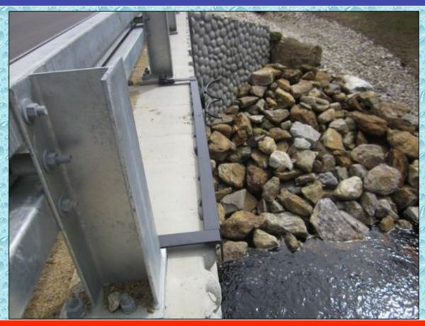
This installation used our angle mount brackets which were bolted to the base of the guard rail posts using existing bolts. The angle mount brackets allow for adjustment over time if the stream flow changes.
