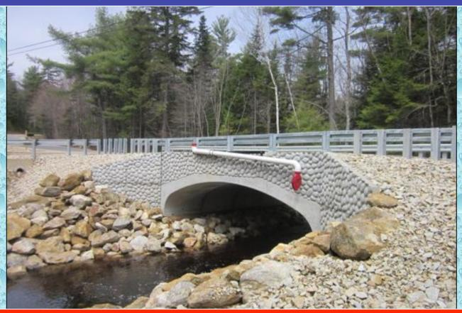
This bridge-mount was installed on another Town-owned bridge and used the existing guard rail post bolts to anchor the system in place.
