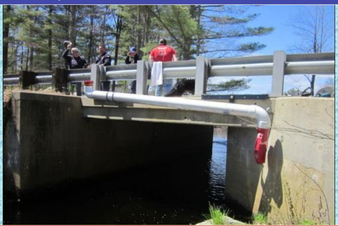
This bridge-mount was installed on State-owned bridge and used the existing guard rail post bolts to anchor the system in place.
