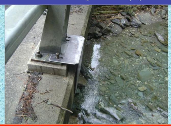
The brackets were fabricated to bolt onto the base of the guard rail posts where they attached to the bridge deck.
