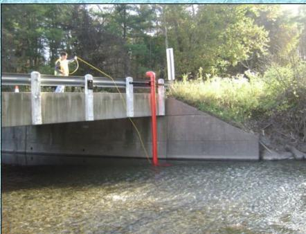
This bridge-mount was installed on another County-owned bridge in Hudson County, New York and used the existing guard rail post bolts to anchor the system in place.
