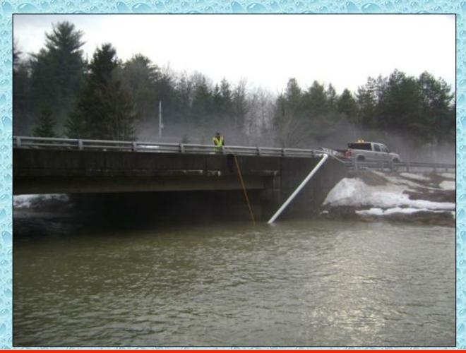
Once in place on the rocky stream bottom, the dry hydrant is ready for use.
