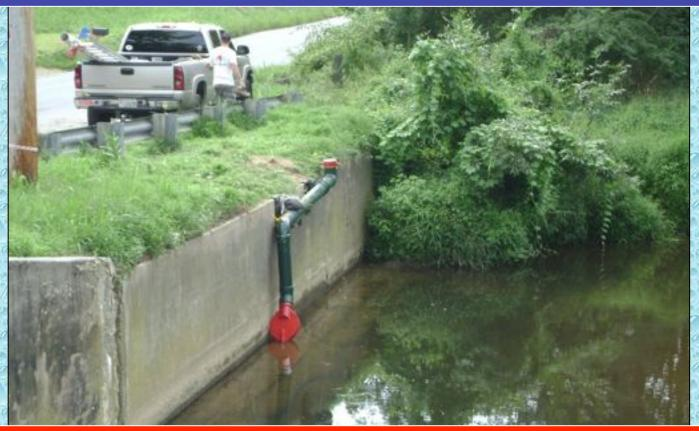
This swiveling standpipe replaced a fixed, dry hydrant that was damaged during flooding. The special "L" shape design was needed to clear a concrete shelf area under the water.
