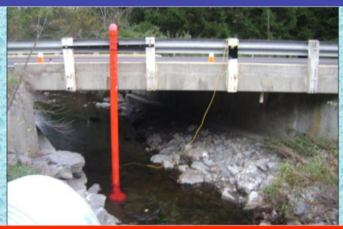
Like the other swiveling standpipes, once deployed...the suction strainer rests on the stream bottom and supports the weight of the standpipe.
