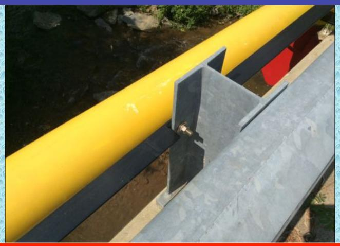
This design is bolted to the stream side of the guard rail posts using existing holes in the posts or by drilling new holes.
