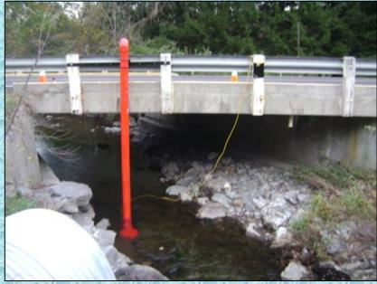
This installation on a County-owned bridge was anchored to the bridge using the existing guard rail structure.
