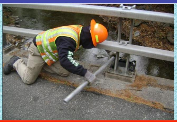
A New York DOT worker ensured proper tension on each bolt during the installation process.
